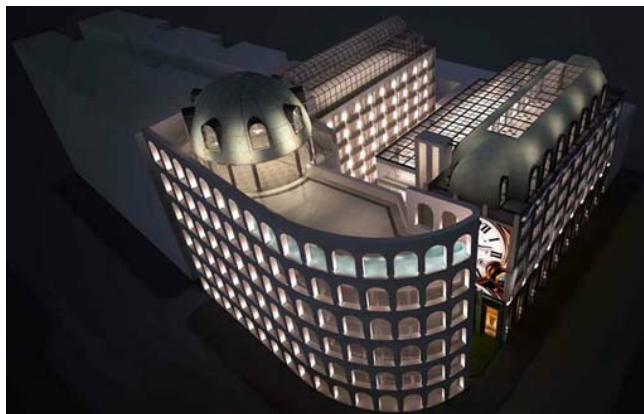
©Shanghai Jiangning Road Power Plant Alteration by STDesign
